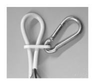
Install the carabineer in the eye bolt previously fixed on ceiling.
